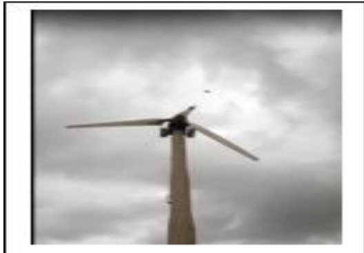
Figure : Structure inspection
