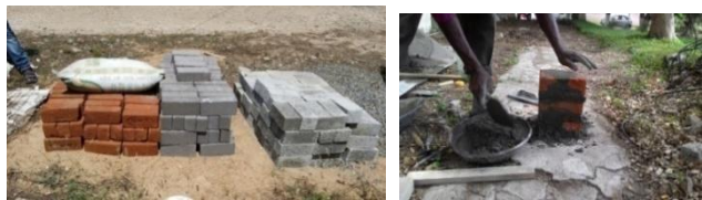
Fig.1 Types of bricks Fig.2: Casting of normal brick prism
