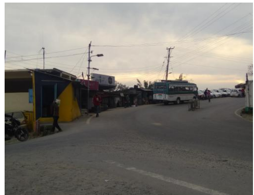
Fig.4. Absence of traffic light and traffic signals at Mehli junction
