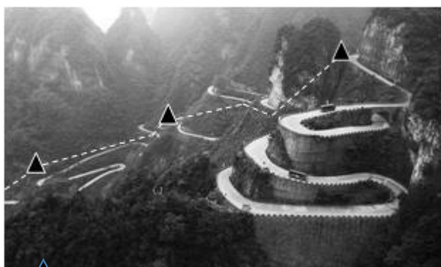
EFL (Environment Friendly Link) stations along the route Optic fiber cable (underground)
