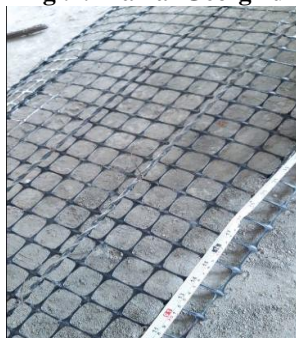
Fig .3. Combination of GFRP and Geo-grid reinforcement
