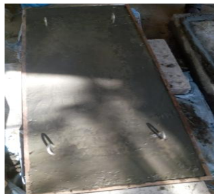
Fig .4. FGRCS slab mould filled with concrete
