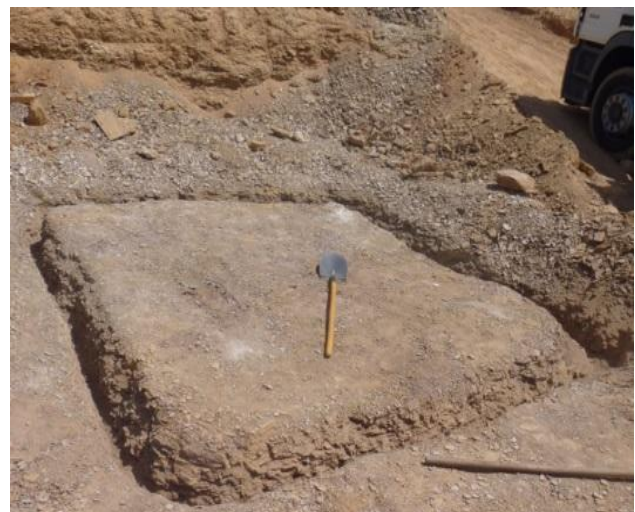
Fig. 6. Preparation of footing location
