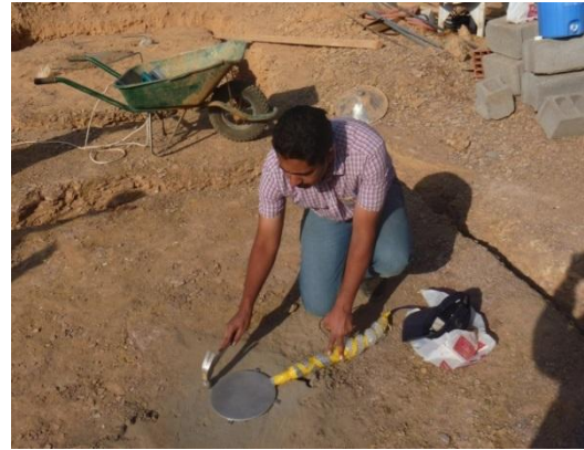
Fig. 8. Earth pressure cell installation
