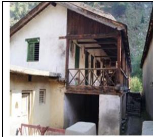
Figure 14: Stilted house built using stone and timber, and then plastered
