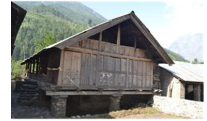
Figure 15: Stilted house built using stone for the lower floor, while timber for wall and floor
