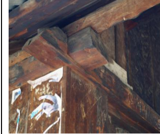
Figure 17: Joinery details
