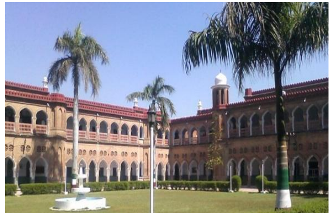
Fig. 1. STS High School (North-East Wing)
