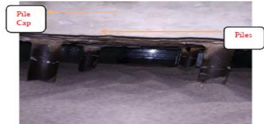
Fig 3 Pile Foundation (piles embedded in soil strata)
