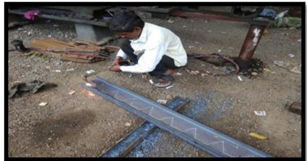
Fig. 5. Cutting of the beam
