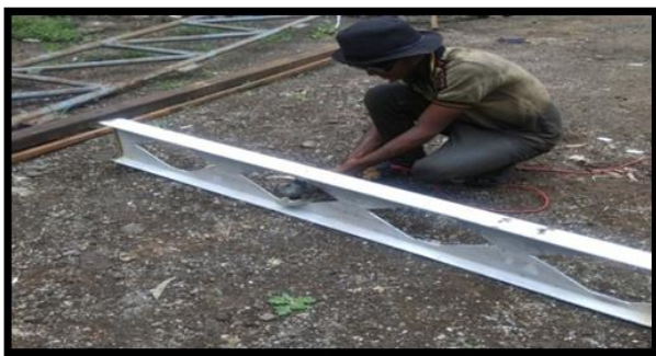
Fig 8. Grinding of a Castellated Beam
