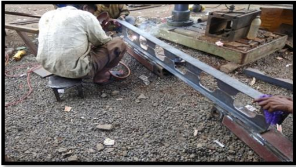
Fig 7. Welding of Castellated Beam
