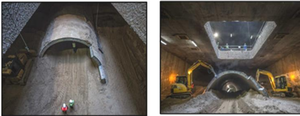
Fig. 16. Excavate to half of the tunnel and removing the tunnel segments, [6]
