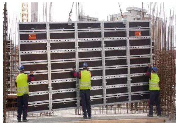
Fig.1: Placing of prefabricated structures around The steel reinforcement
