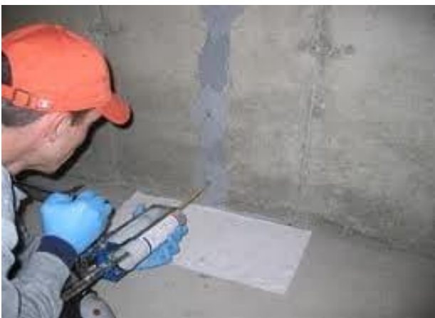
Figure 2: Repair of cracks by Epoxy-injection method [24]
