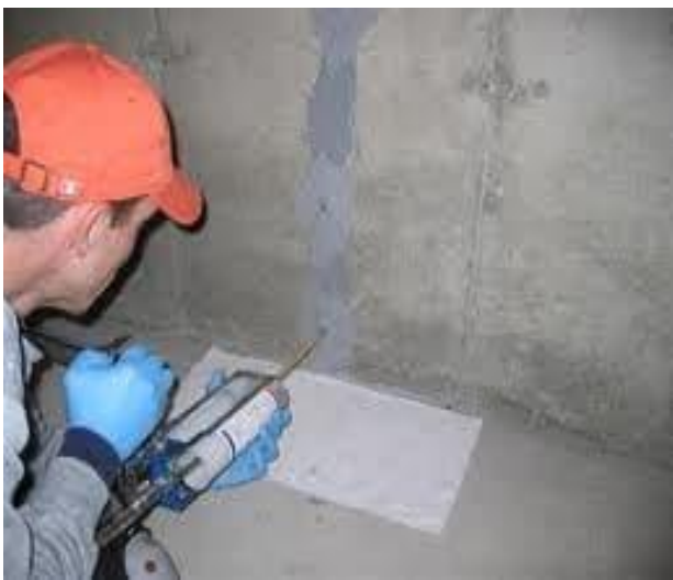
Figure 2: Repair of cracks by Epoxy-injection method [24]
