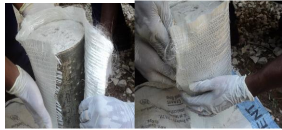
Fig.3 Applying of fiber sheet
