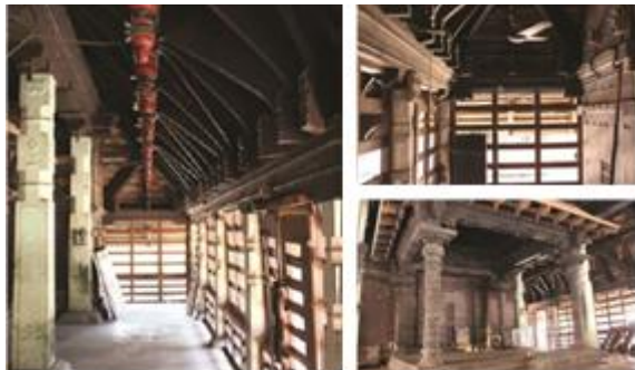
Fig.7. Maximum light from both the sides of Koothambalam (Ventilation around the passage)
