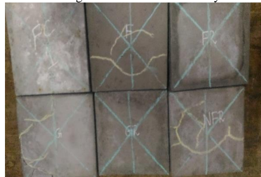
Fig. 7. Typical crack pattern on top surface of panels
