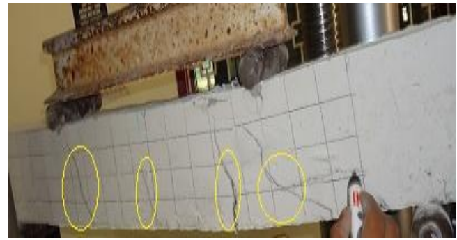
Fig. 3 Cracking pattern of beam
