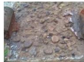
Fig. 9. Rail seat abrasion [22]
