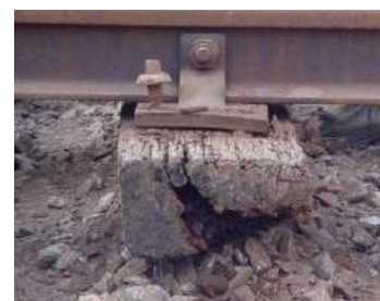
Fig. 5. Decompose due to fungus (9)
