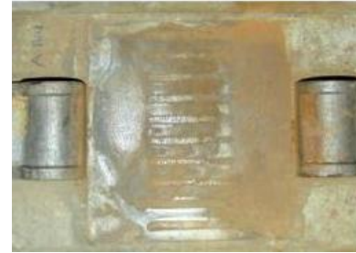
Fig. 24.Rail seat covered by a steel plate after 10 million cycles [49].
