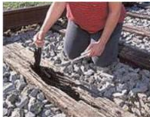
Fig. 7. Attack by Termites [13]
