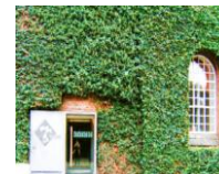
Fig.1 : Direct Green Facade- Self-climber plants planted at the base of the building.
