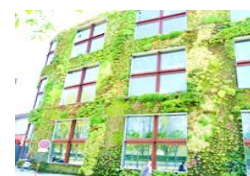
Fig.3 : Green Walls/ Living Walls: Living wall systems also known as green walls, are constructed through the use of modular panels, which contains its own soil or other artificial growing mediums, for example foam, felt, perlite and mineral wool, based on hydroponic culture.
