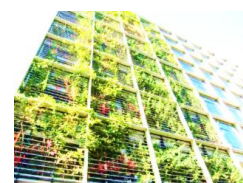
Fig.2 : Double skin vertical/indirect green façade.- Plants grown on another layer apart from the wall.
