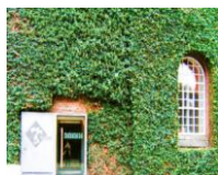
Fig.1 : Direct Green Facade- Self-climber plants planted at the base of the building.
