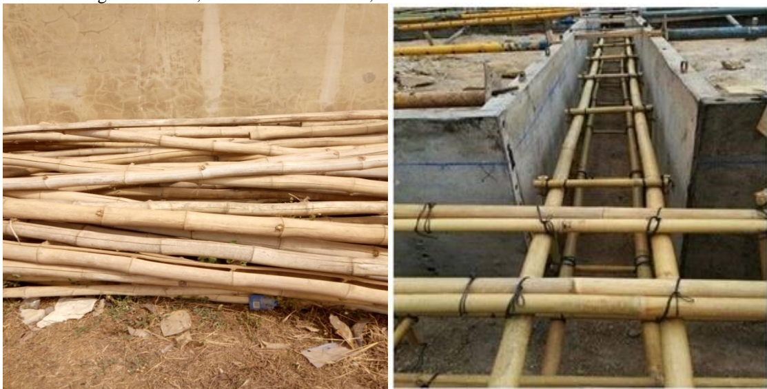
Figure 2: Stocks of Bamboo and its arrangement in a concrete beam. Source: engineering society.com
