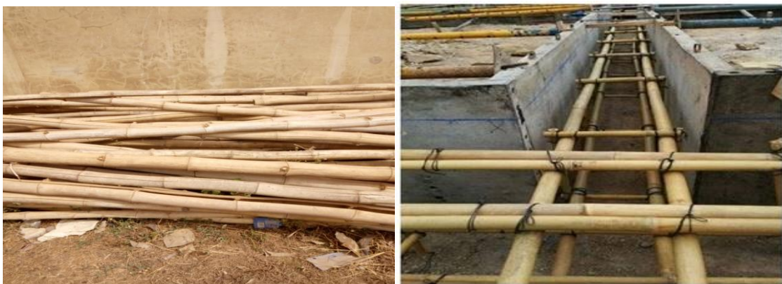
Figure 2: Stocks of Bamboo and its arrangement in a concrete beam. Source: engineering society.com
