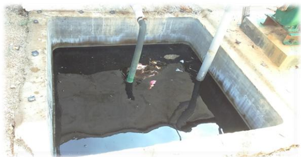
Fig 1 Landfill leachate collection tank
