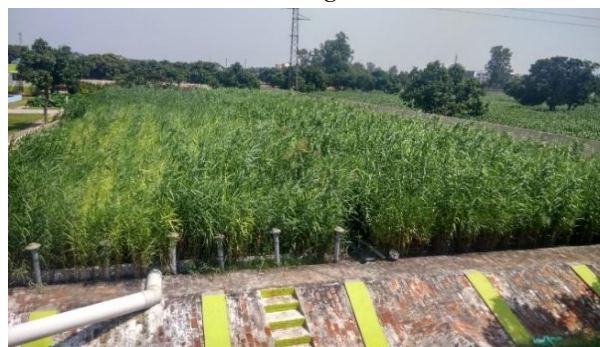
Figure 3: View of Vertical Flow Constructed Wetlands at SWINGS WWTP, AMU, Aligarh
