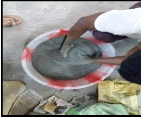
Fig no.3 Mixing of Concrete
