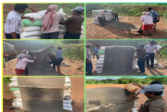
Figure 5 Installation of Sentry post with Sand Bag
