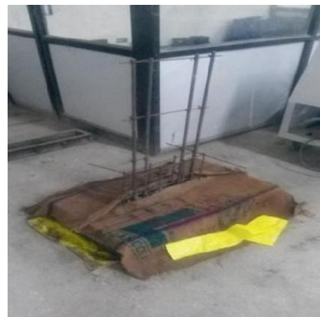
Fig 2. Precast Wall Dowels
