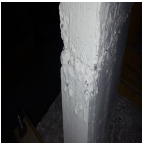
Fig 9. PW3 Cracking
