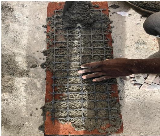
Fig.5 PP Geo-fabric Bed reinforcement
