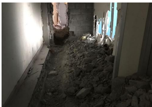
Fig 1: Demolition site from where 8 year old aggregate sample was collected
