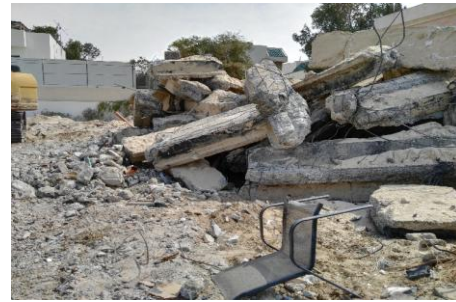
Fig 2: Demolition site from where 16 year old aggregate sample was collected
