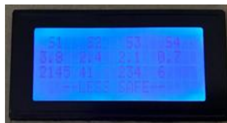
Figure 6: 'Less safe' Level Screen
