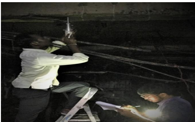
Fig. 2. Rebound hammer test
