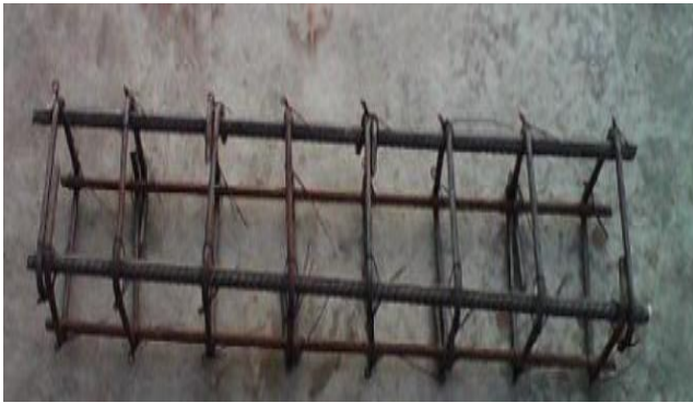
Fig.2: Reinforcement Details of Beams
