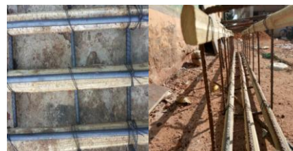
Fig 3: Bamboo reinforcement
