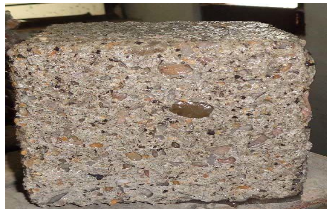
Acid Attack on Concrete Cube
