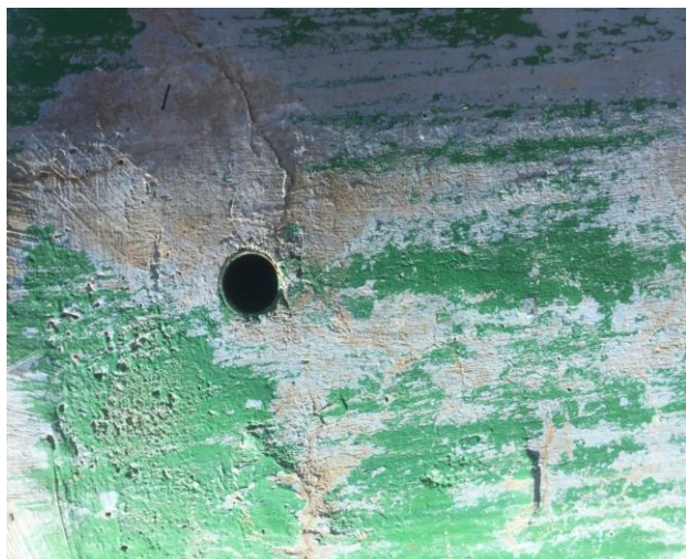
Fig.2. Column of Station G-4, 1.6 inch diameter throughout hole
