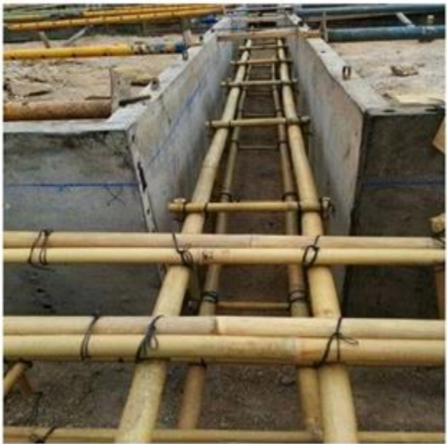
Fig. 2. Bamboo arrangement in a concrete beam. Source: engineering- society.com
