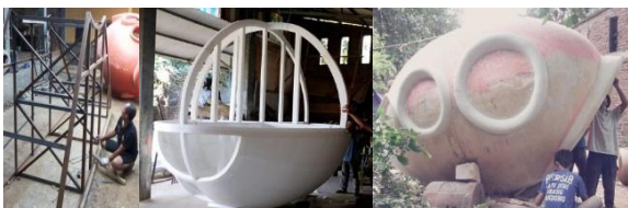
Fig 2: The construction of three-dimensional work electrically welded with elbow-shaped iron materials
