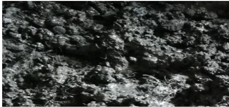
Fig 2: Concrete with plastic fiber (FRCP)
