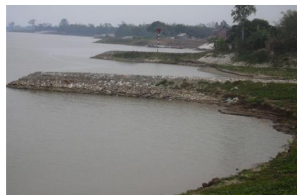
Figure 1. Spur dikes project on the Red river
