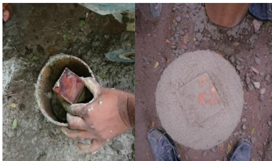
Fig.2: Casting of CFST Columns
