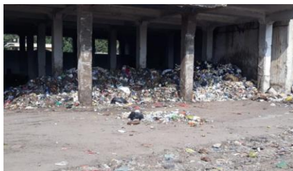
Fig.10: Vijayawada- Autonagar transfer station
