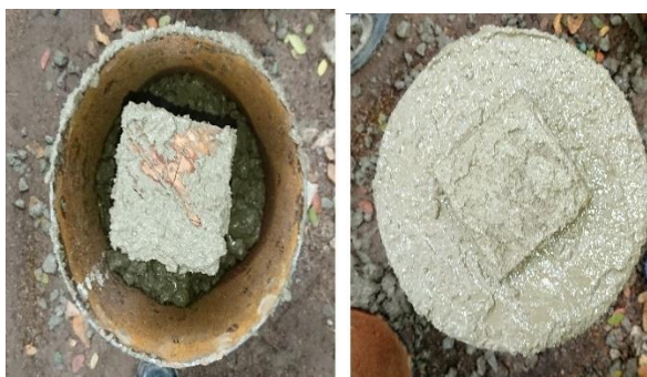
Fig.1: Casting of CFST Columns
