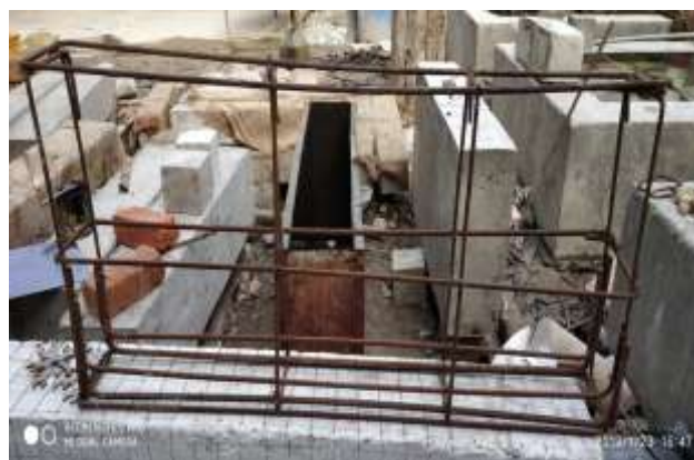
Fig. 4: Casing of steel reinforcement
