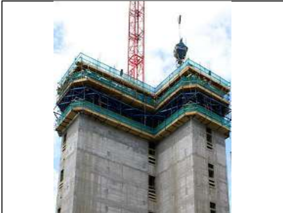
Source: Ramakrishna Venuzia Techno Towers atnear by ANU.(Slip formwork)
