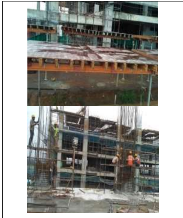
Source: Ramakrishna Venuzia Techno Towers at nearby ANU (Table formwork).
