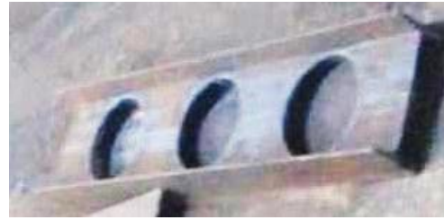
Fig. 3: Cellular beam with three web openings
