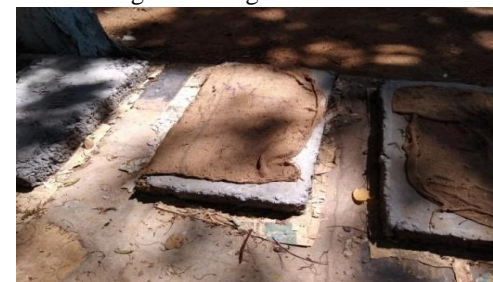
Fig.4 (a). Curing of concrete
