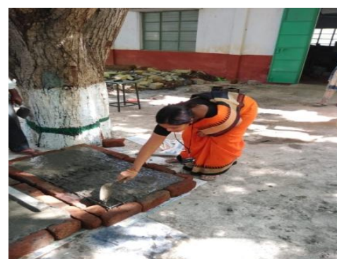
Fig.3. Casting of concrete
