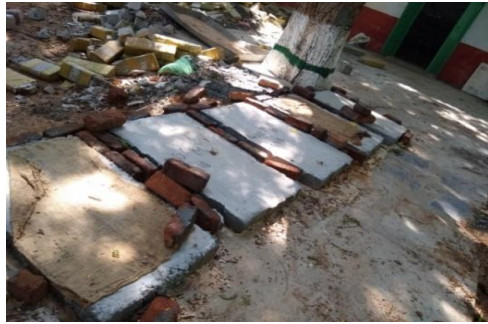
Fig. 4(b). Curing of concrete
