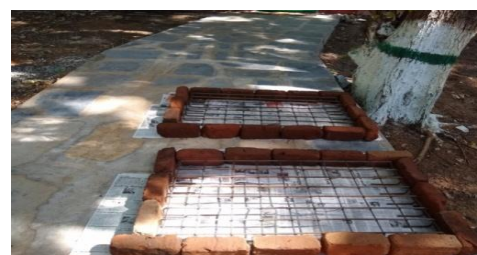
Fig.2. Mould and reinforcement arrangement before casting
