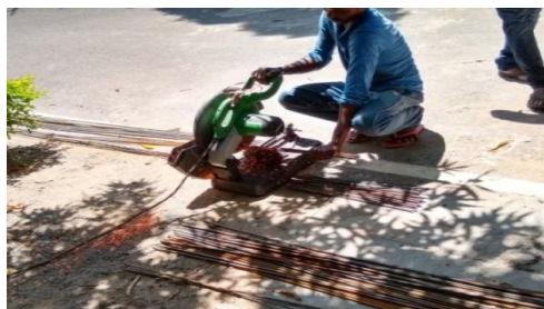
Fig.1. Cutting of steel rods
