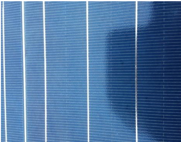
Figure 1b: Shading due to Building
