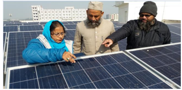
Figure 2b: SPV Panels on Roof Top of Integral University
