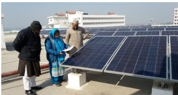
Figure 2a: SPV Panels on Roof Top of Integral University
