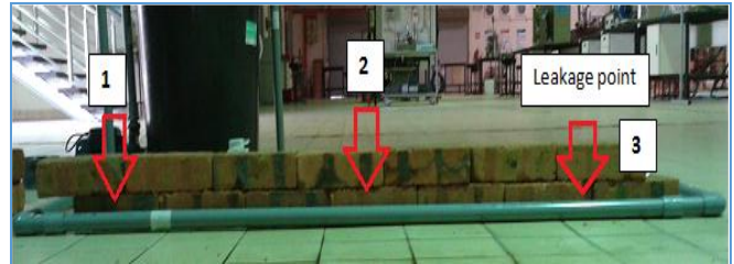
Fig. 5: Leaked pipe and the leakage point
