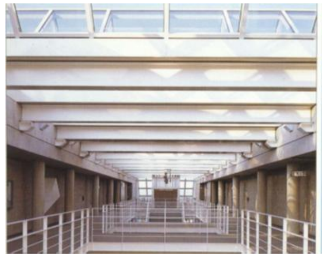
Fig. 2 Daylight Entering Building
