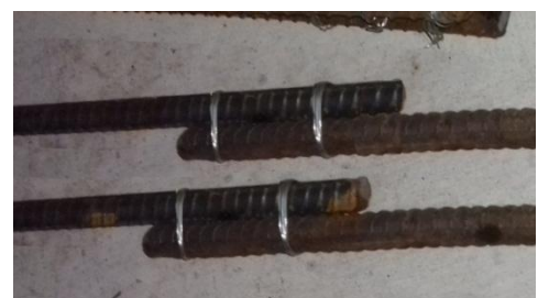
Fig. 4: Lapping of rebar
