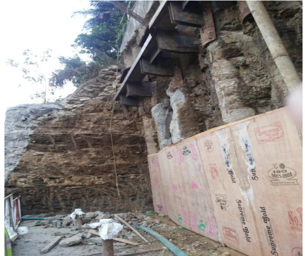
Figure.3 Commercial plywood fixed on wooden frame constructed for skin wall
