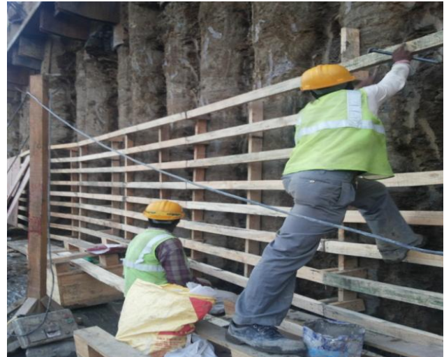
Figure.2 Wooden framing for skin wall construction
