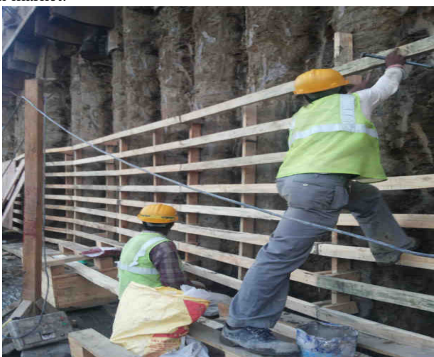
Figure.2 Wooden framing for skin wall construction
