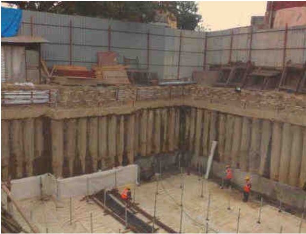
Figure1. Plume concrete wall constructed for fixing waterproofing membrane at Project site
