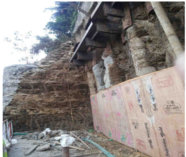
Figure.3 Commercial plywood fixed on wooden frame constructed for skin wall
