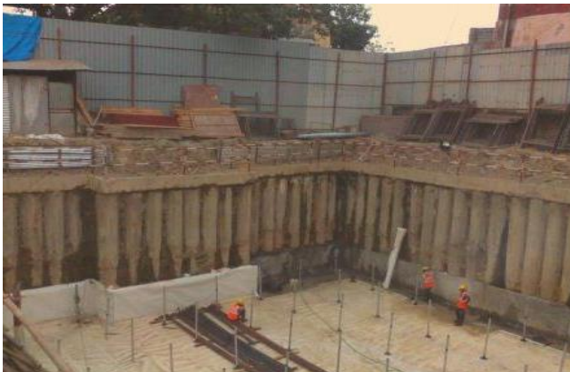
Figure1. Plume concrete wall constructed for fixing waterproofing membrane at Project site
