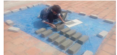
Fig. 8 Casting of Brick
